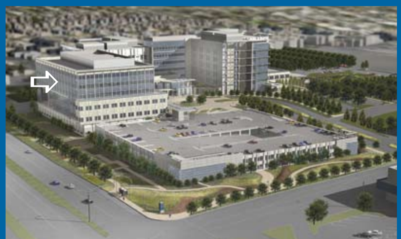
Aerial view of the new hospital and the proposed Professional Office Building.
