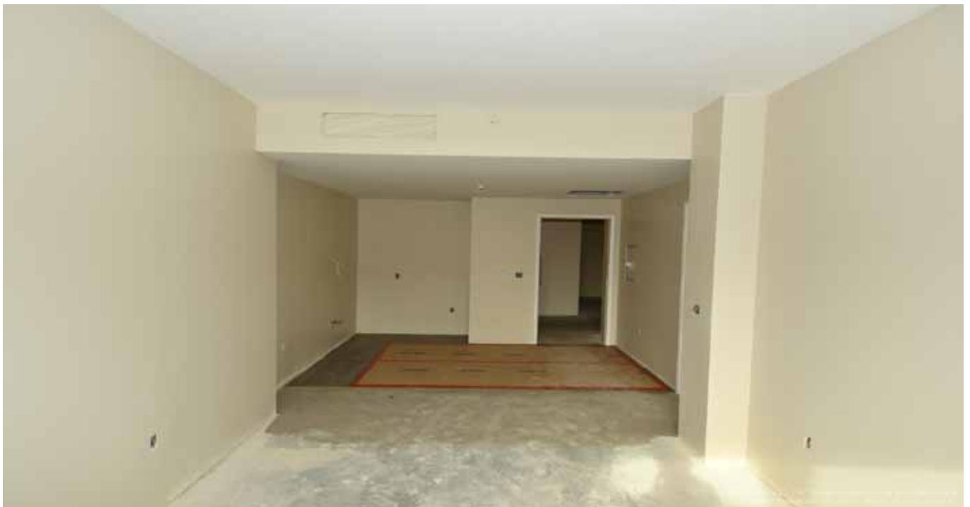
Interior unit painted, Flooring installed waiting for kitchen casework and carpet
