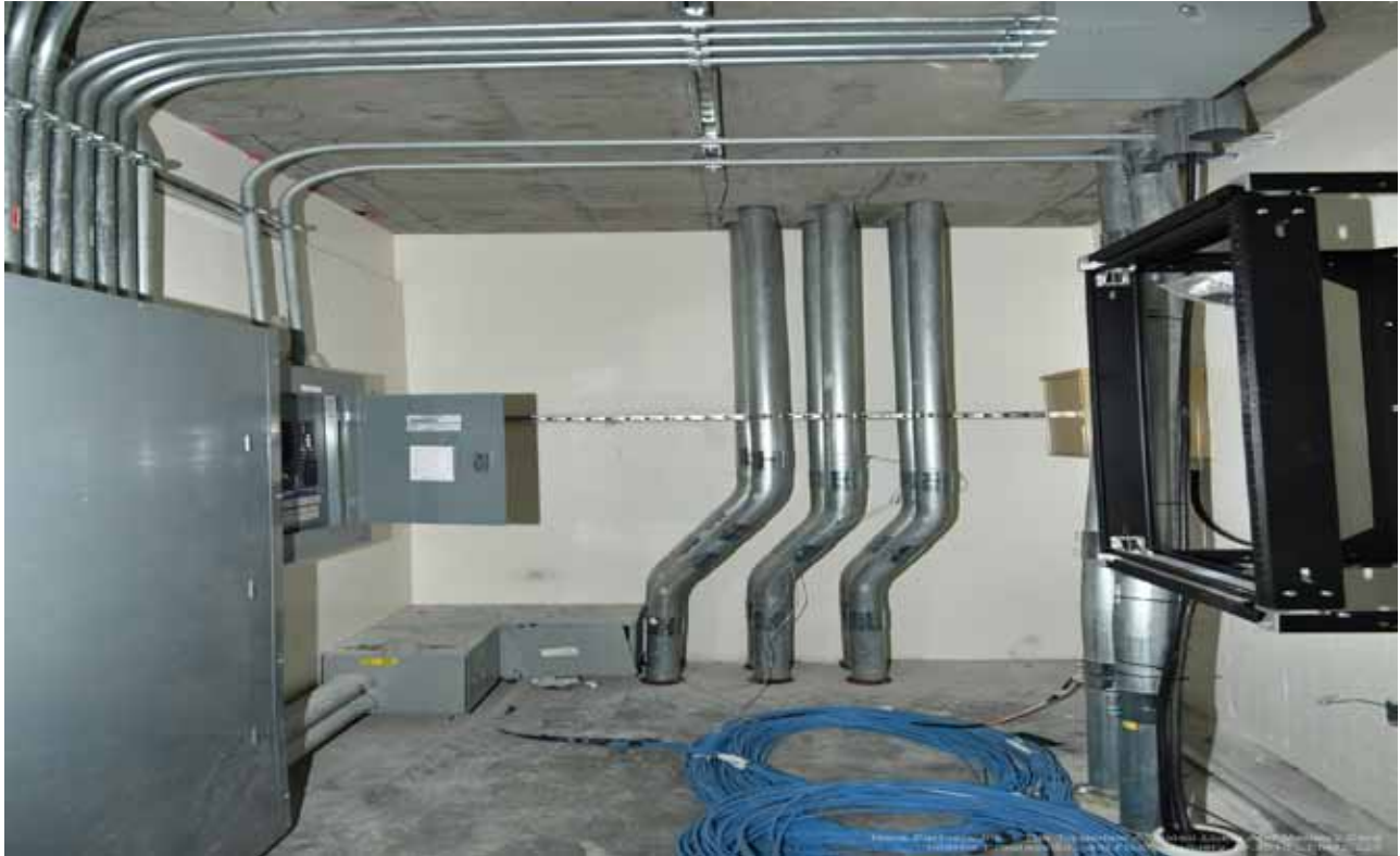
Floor 2 Electrical rooms near completion
