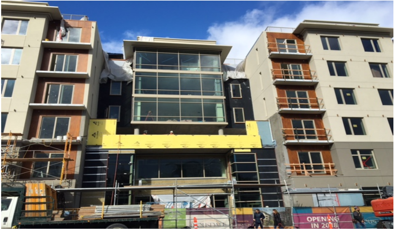
Main Entry glazing installed waiting on final finishes
