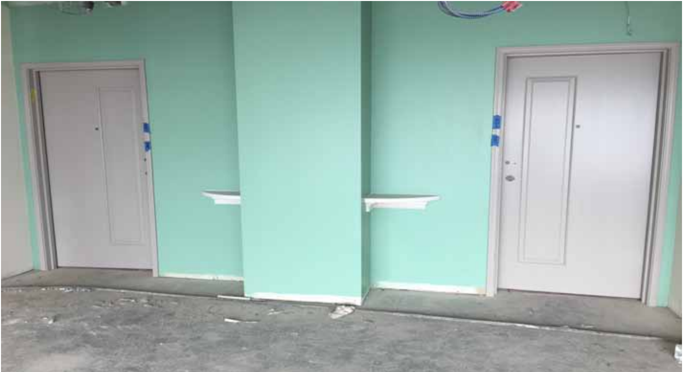
Floor 2 Residential unit entry
