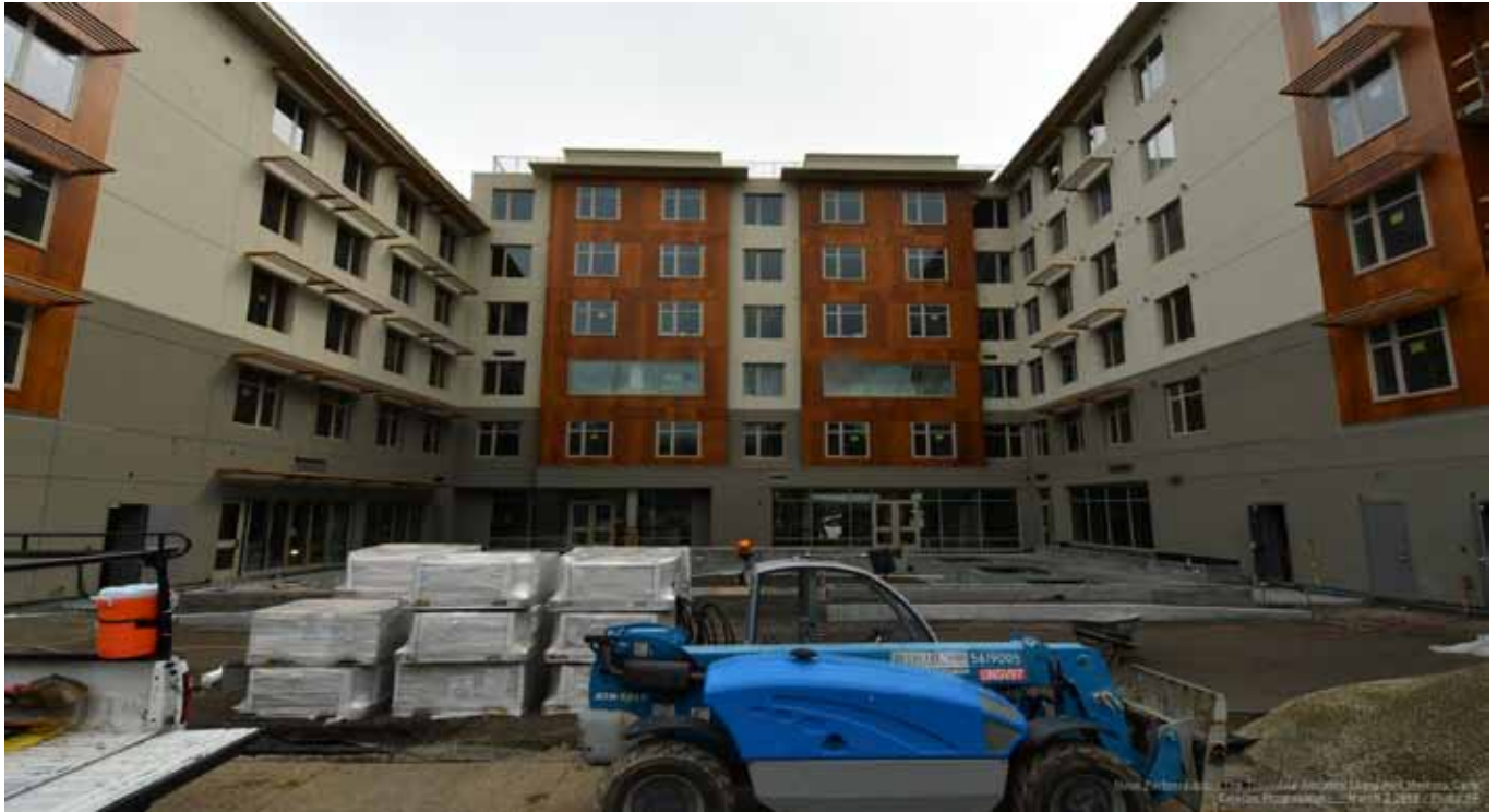
Courtyard Pavers being installed. Exterior skin complete
