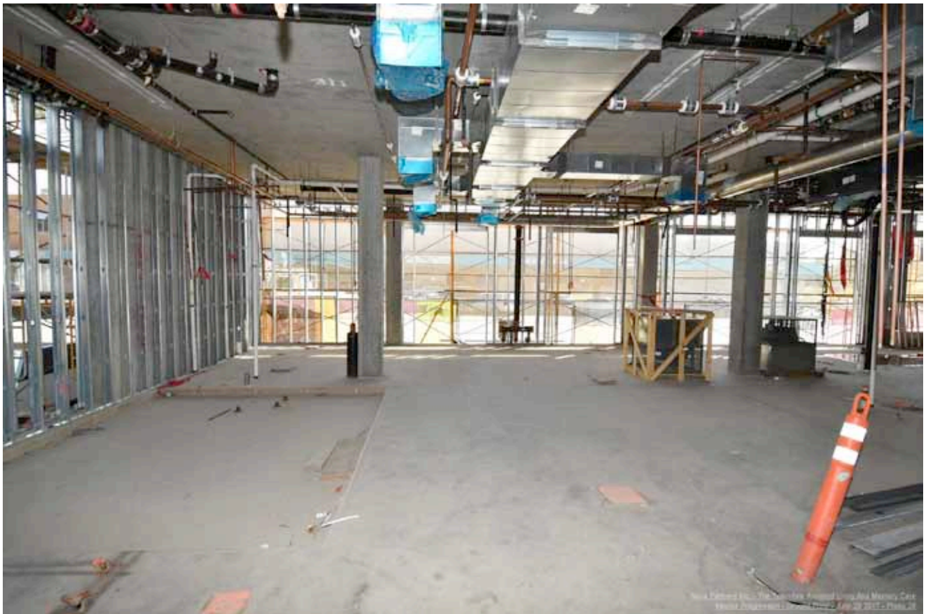
Floor 4 overhead M/E/P systems installation underway. Exterior framing complete.
