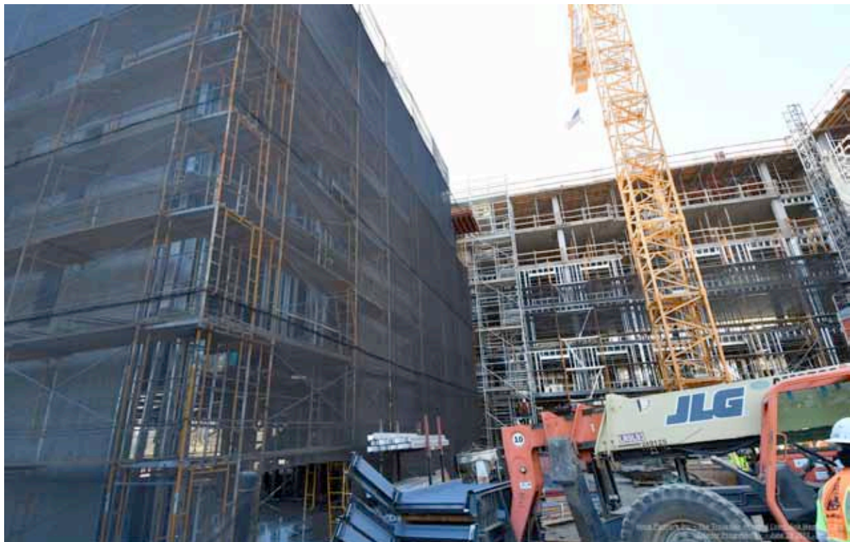
Central Courtyard looking to the South. Exterior framing underway approx. 90 % complete.
