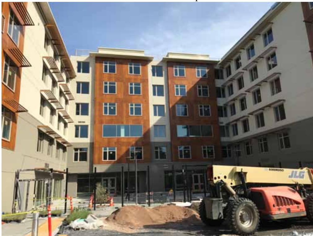
Courtyard planting underway
