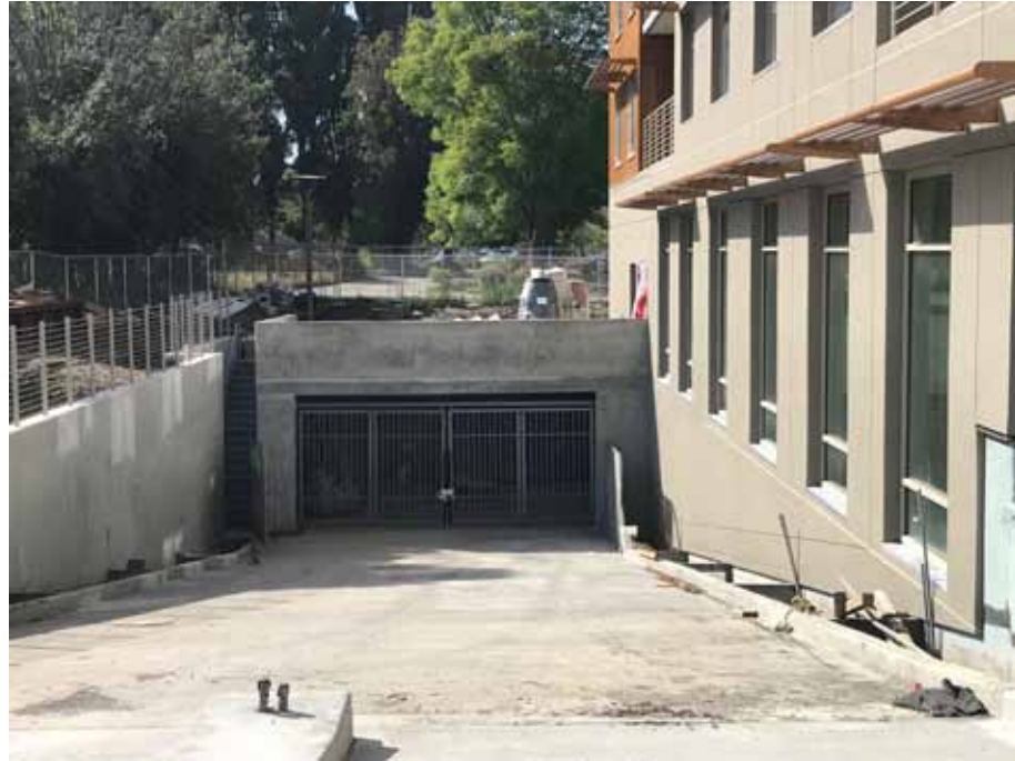
Basement ramp poured out with garage gates installed awaiting final planting
