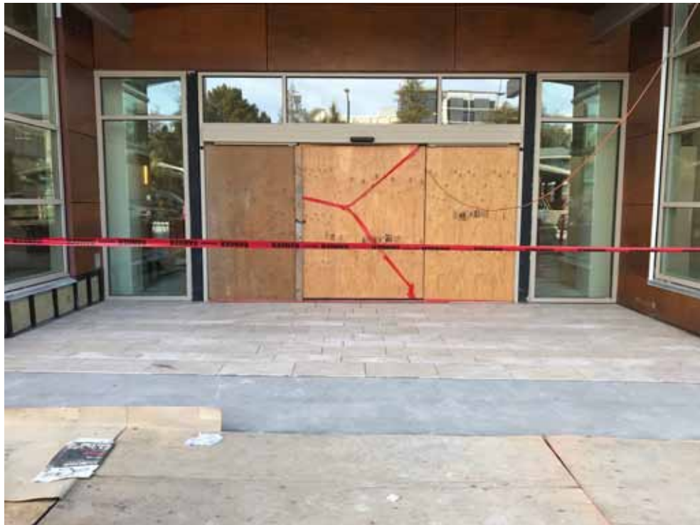
Front Entry completed awaiting wood door install. Stone flooring underway
