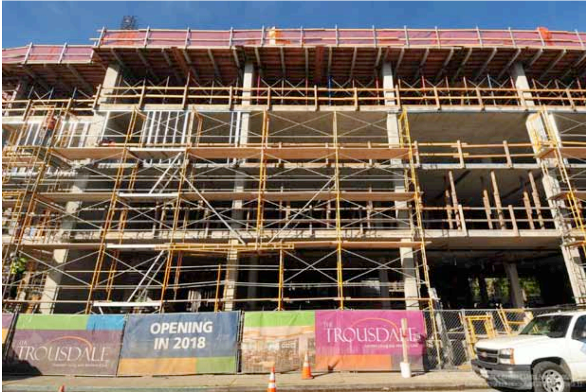
South Elevation with Scaffold up and Floor 3 exteriors framing underway.
