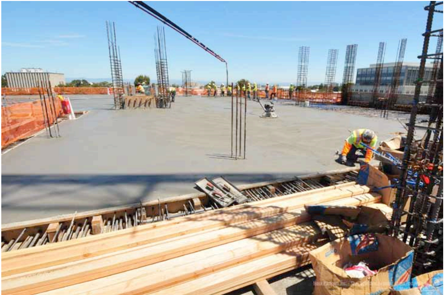
Floor 5 West Slab deck just being poured.
