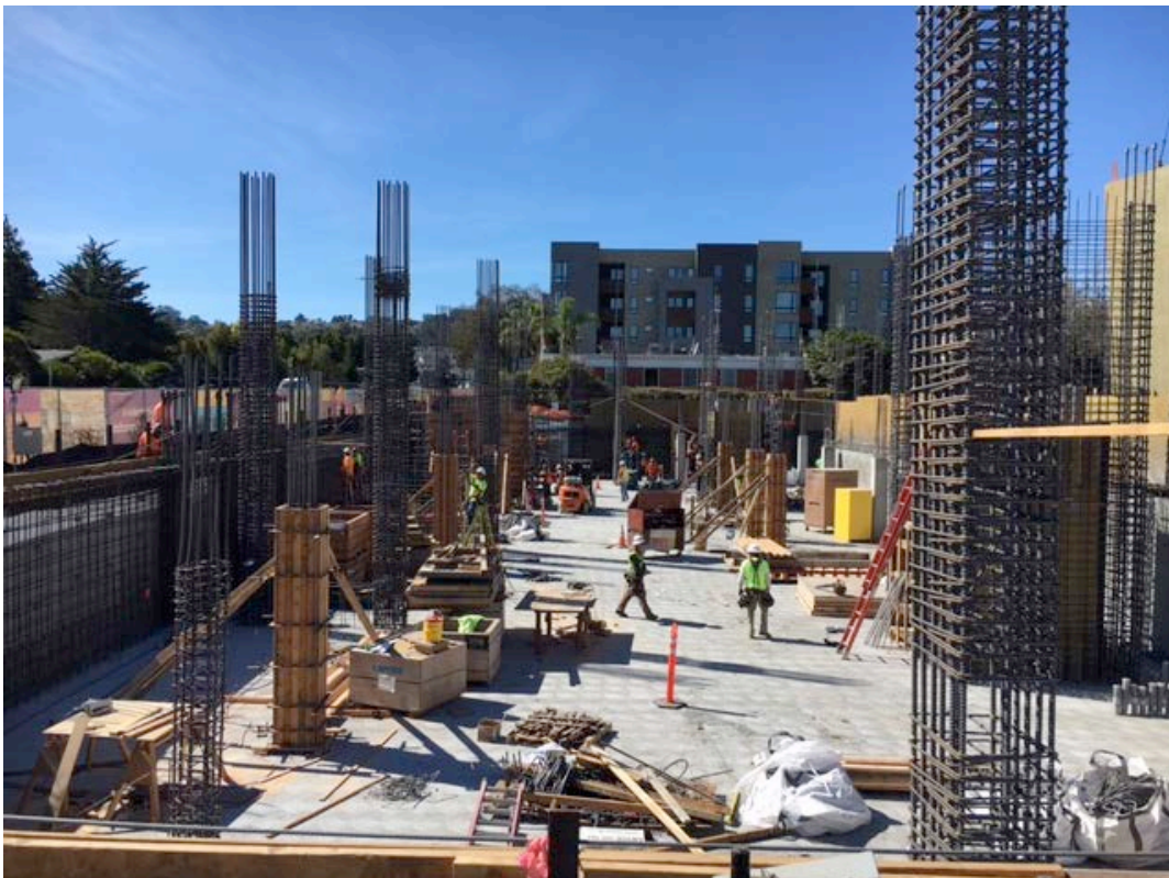
(10/6/16) Basement looking West
