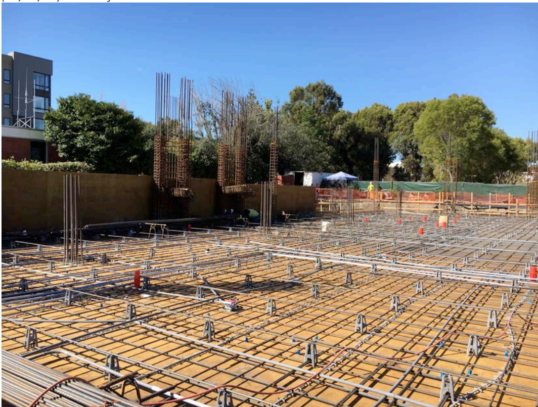
(10/26/16) Ground floor rebar and conduit installation
