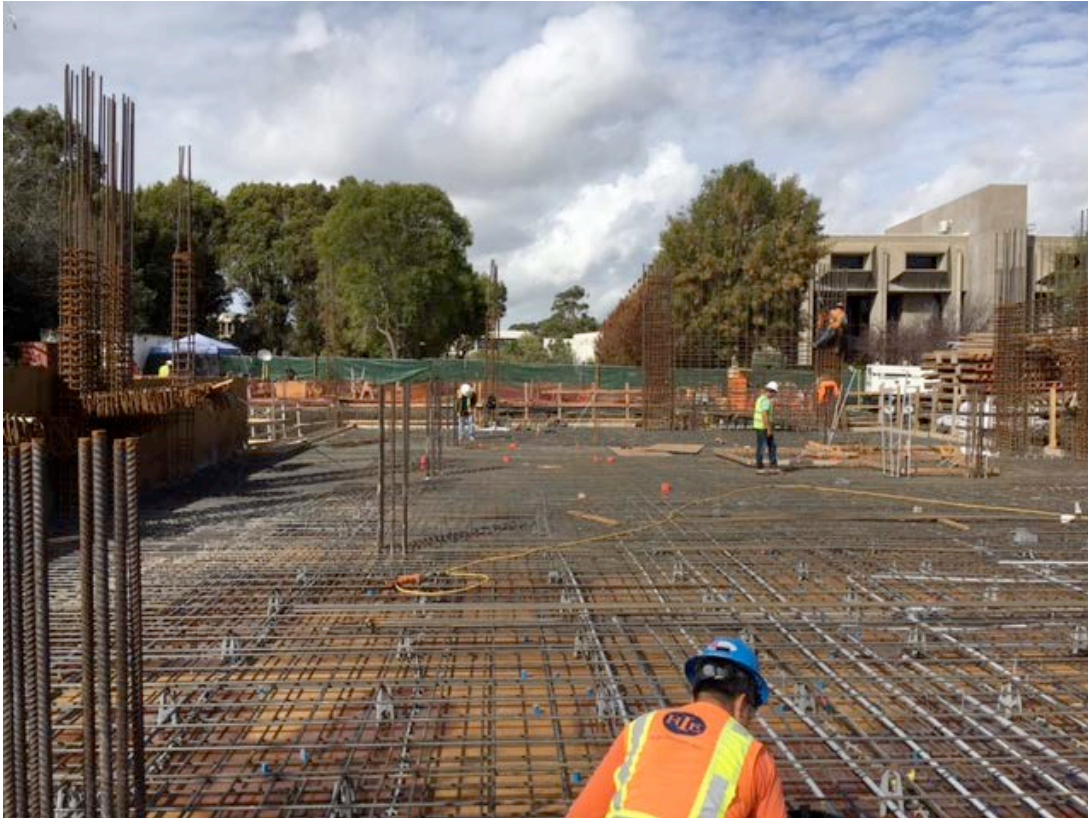
(10/31/16) Ground floor rebar and conduit installation
