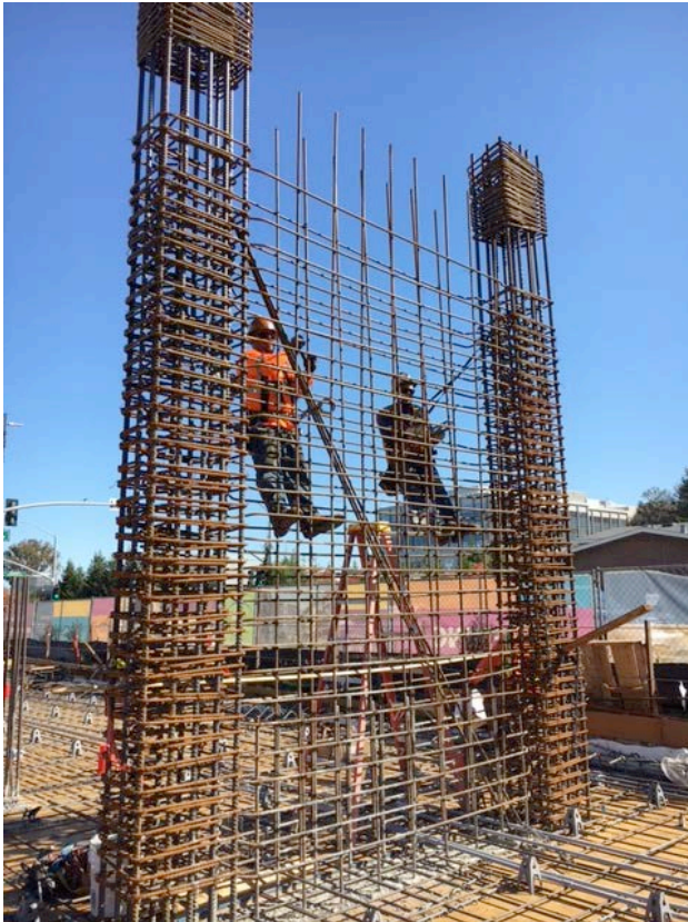
(10/26/16) Ground floor Shearwall rebar installation
