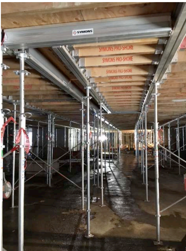
(10/18/16) Basement Shoring in place for ground floor deck
