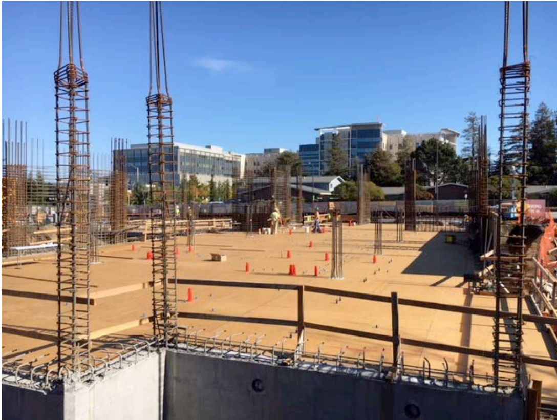
(10/18/16) Ground floor decking looking South
