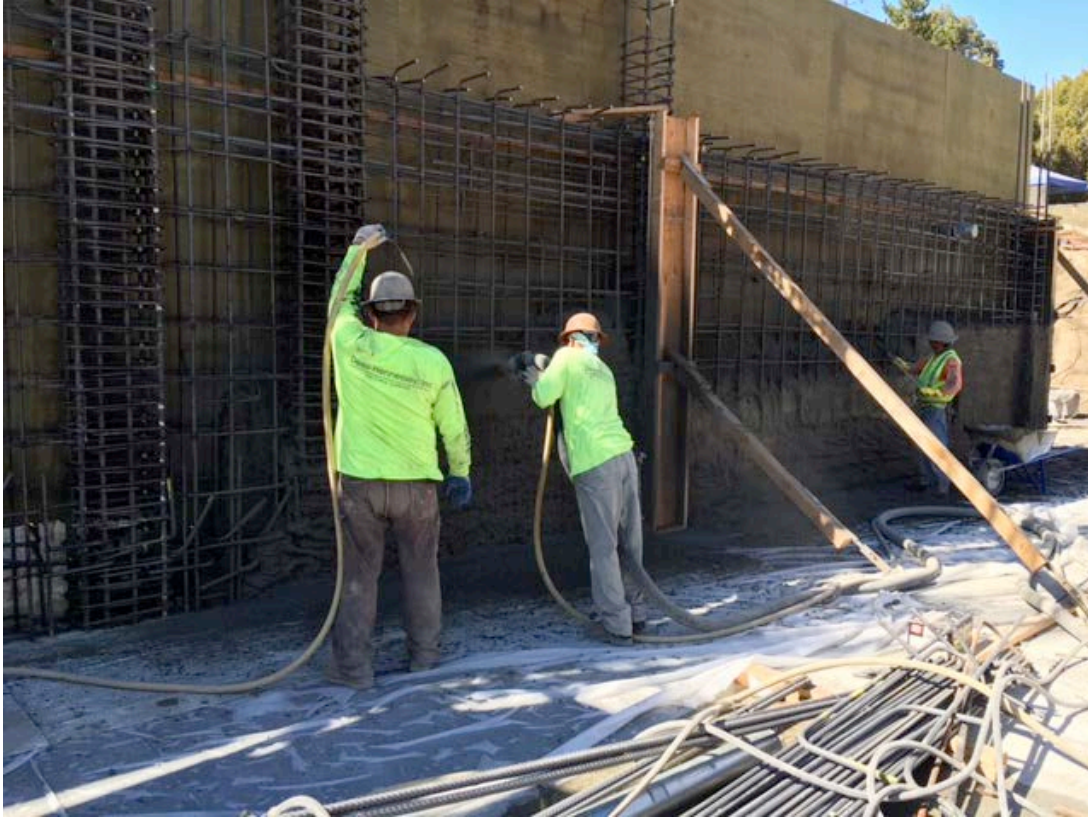
(10/6/16) Shotcrete wall placement in basement.
