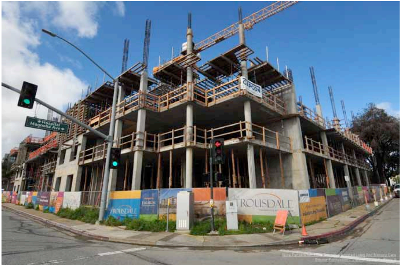
3/31/17 - Fourth floor east slab formwork underway - Looking north/west
