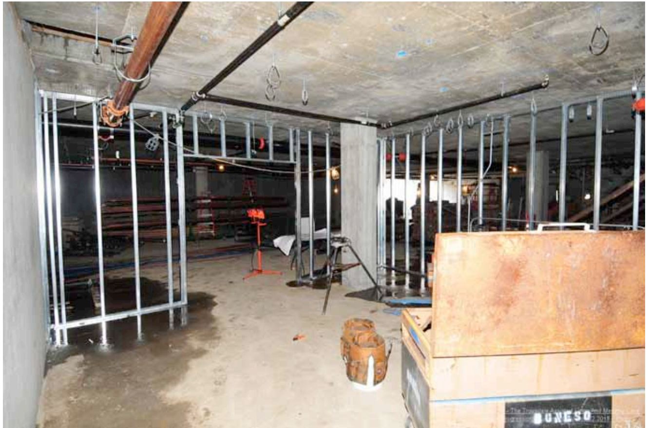
3/31/17 – Basement wall framing/ Plumbing sprinkler pipe rough in
