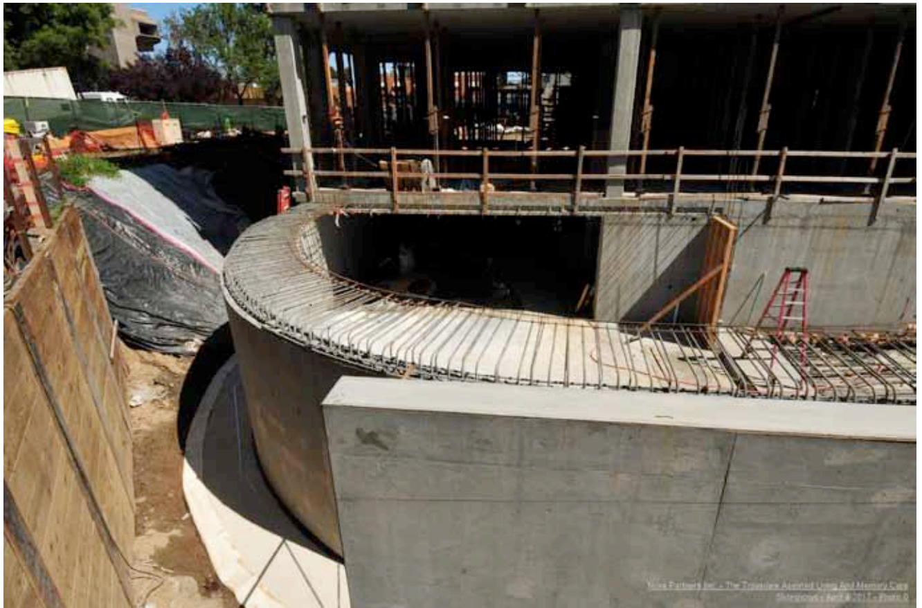
3/31/17 – Basement ramp walls complete. Ready to pour staff patio slab
