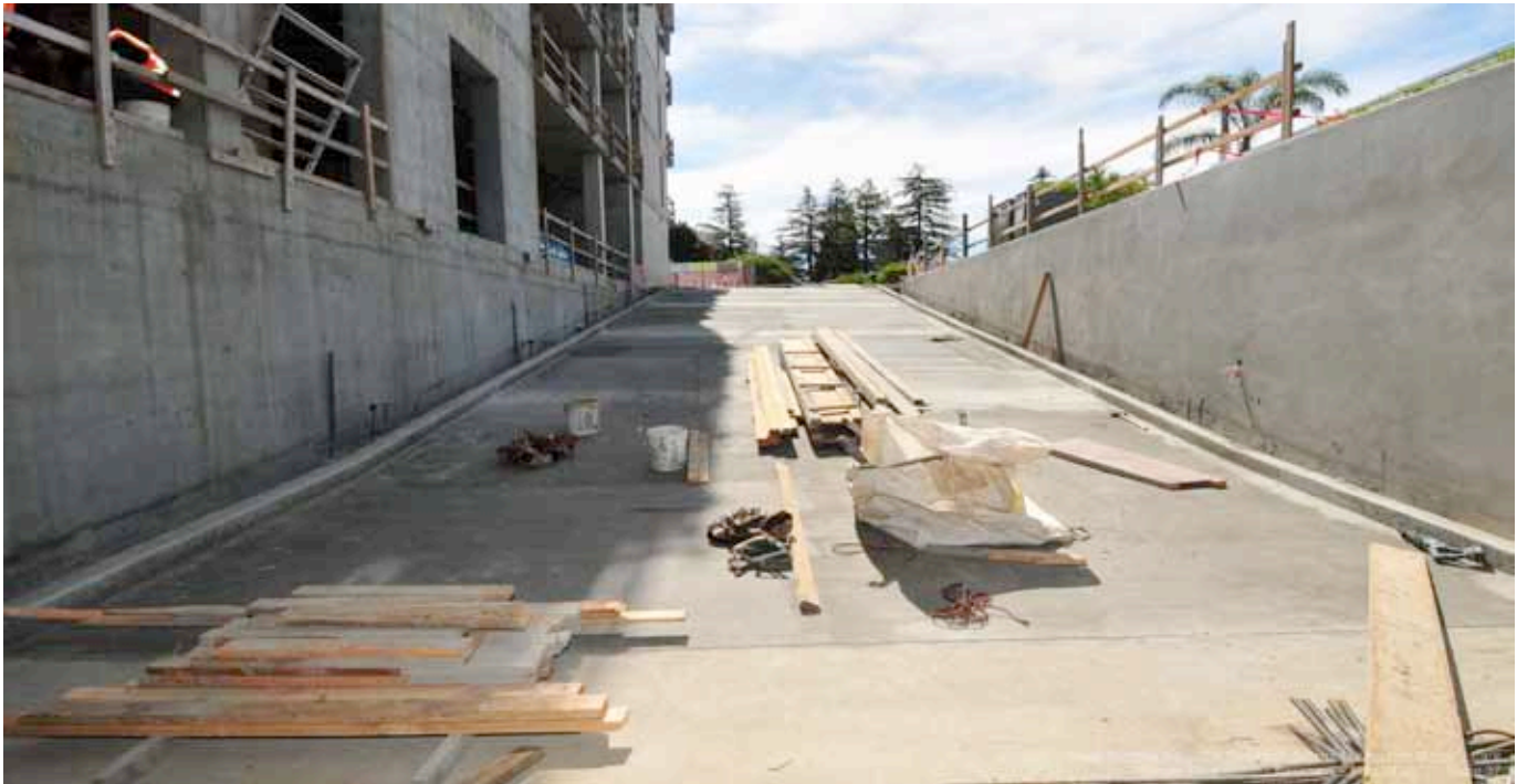
Exterior ramp going down to garage is now complete.
