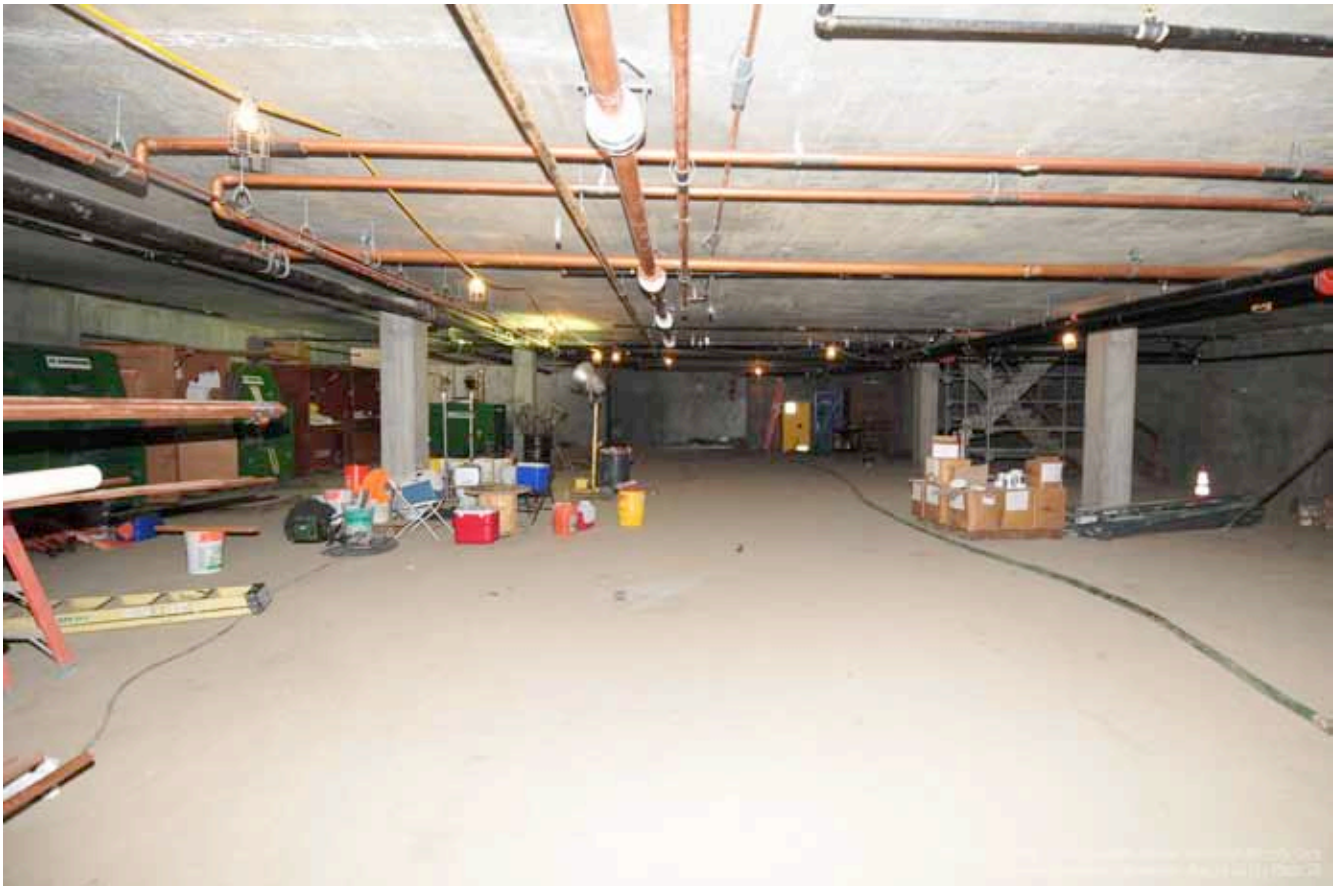
Basement plumbing installed and approximately 90% complete.
