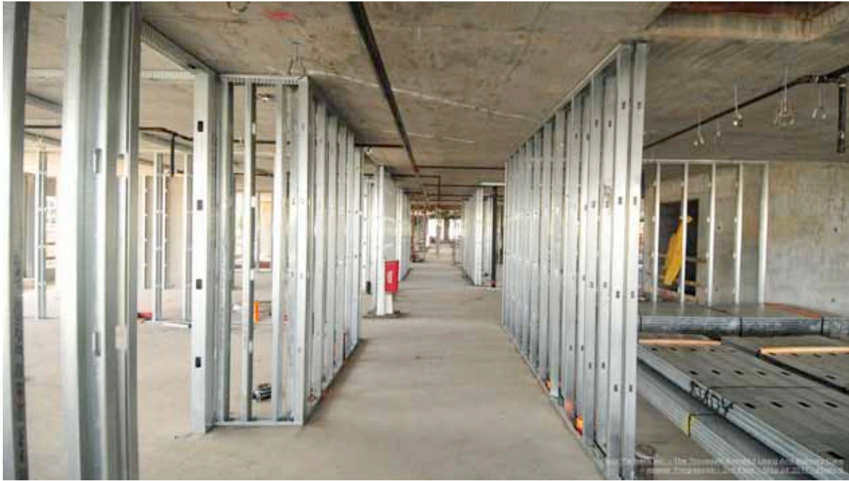
Floor 3 interior framing in progress.
