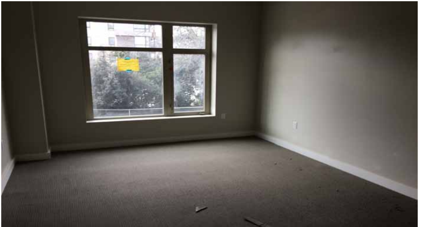
Residential unit carpet installed
