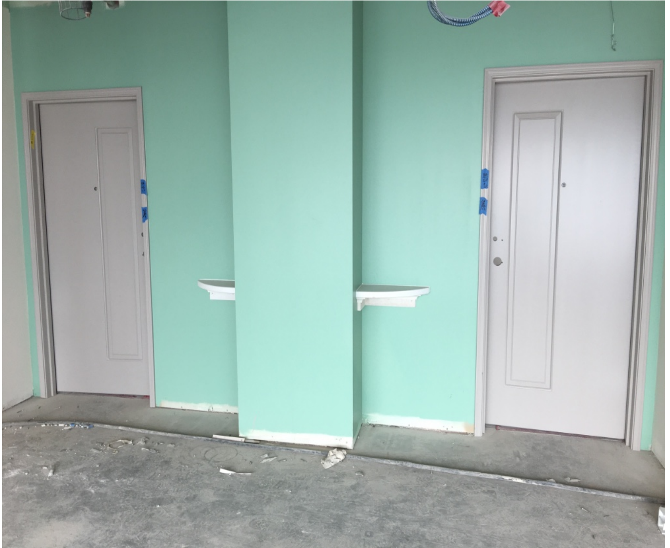
Floor 2 Residential unit entry
