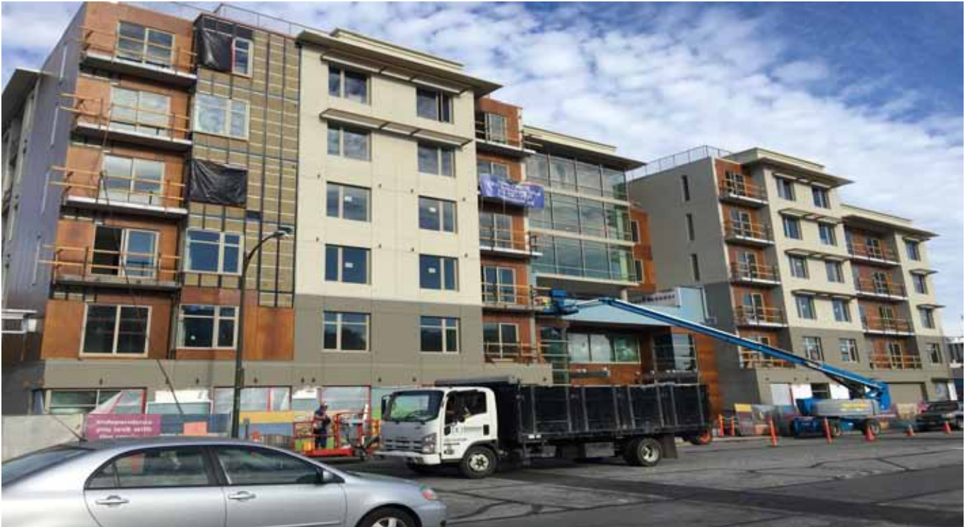
Main Entry/South Elevation nearing completion
