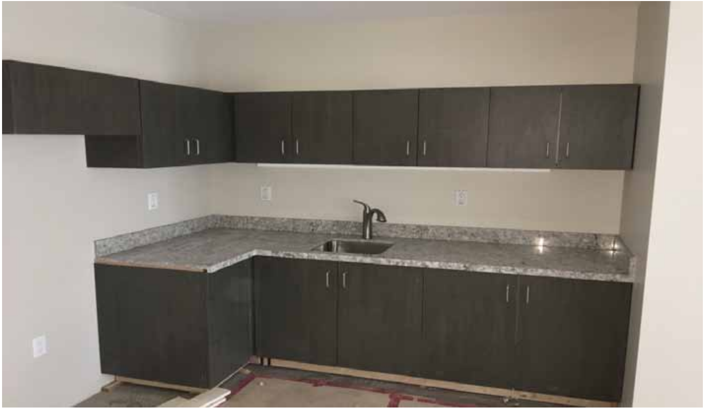
Residential Unit Kitchens installed floors 2 and 3
