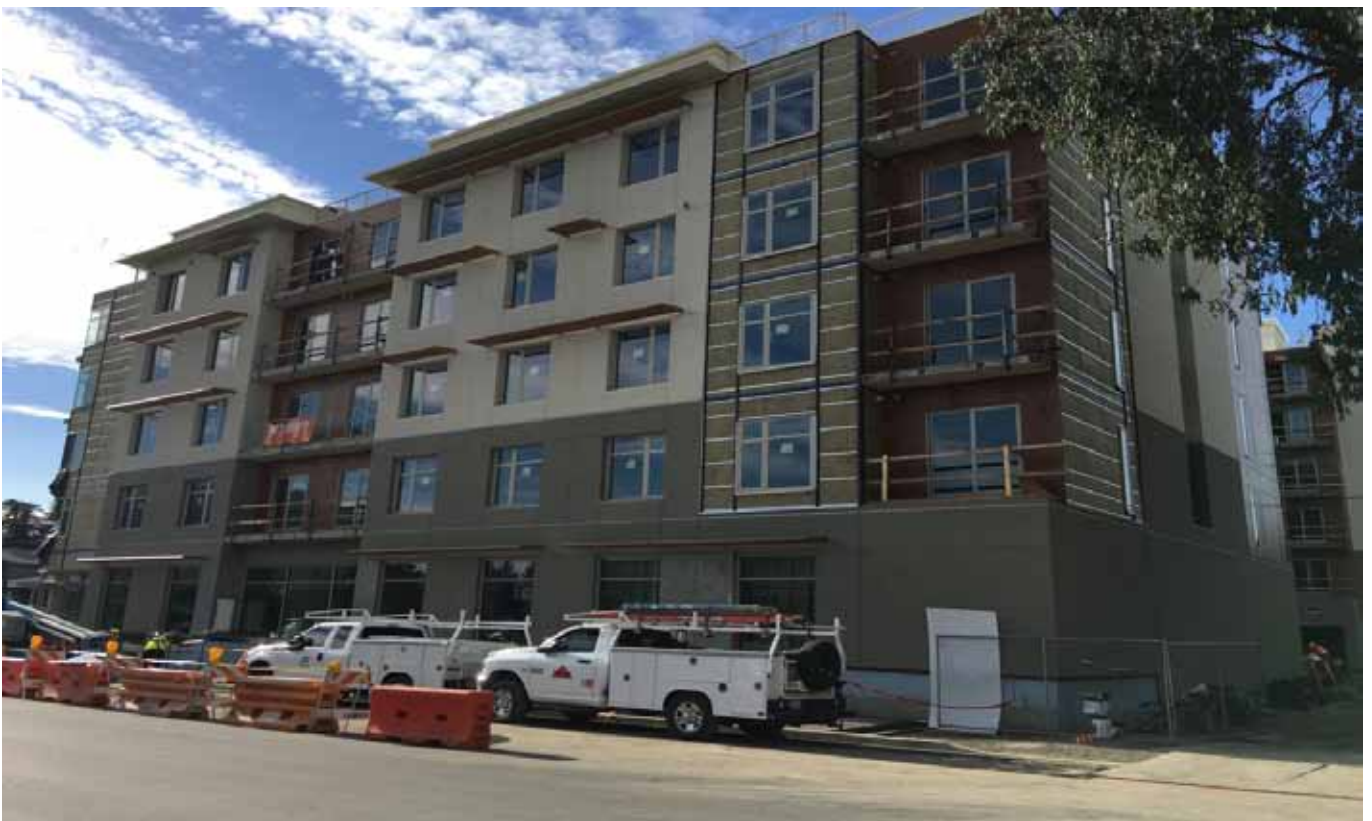
East Elevation with Sun Shades installed
