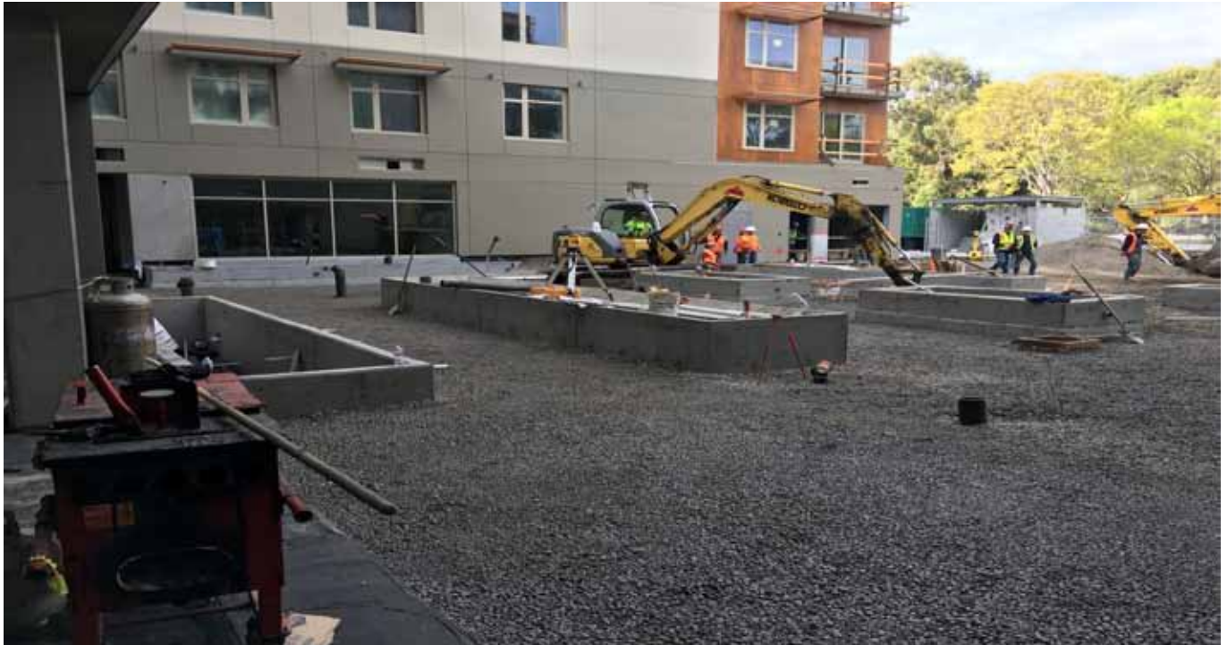
Exterior Courtyard planter walls placed with pavers to begin shortly
