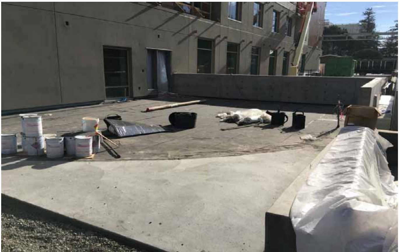
Staff Patio complete waiting on paver installation
