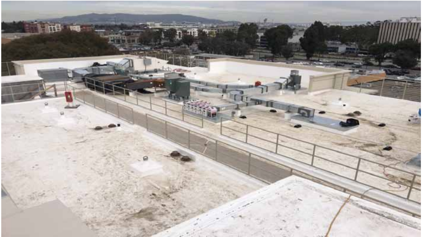
East Roof near completion
